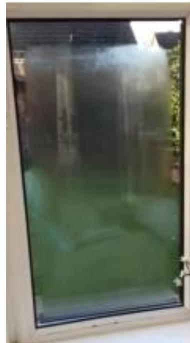
*Figure 1; Example of external condensation on a modern low-e unit. Note clearing around perimeter is caused by heat transfer from inside property passing through the frame.*
