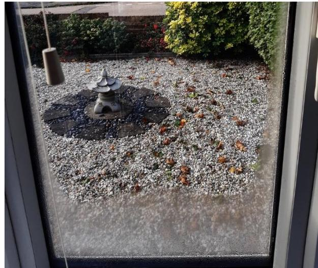
*Figure 2; Example of internal condensation around lower perimeter where glass surface temperature is at it's lowest.*
